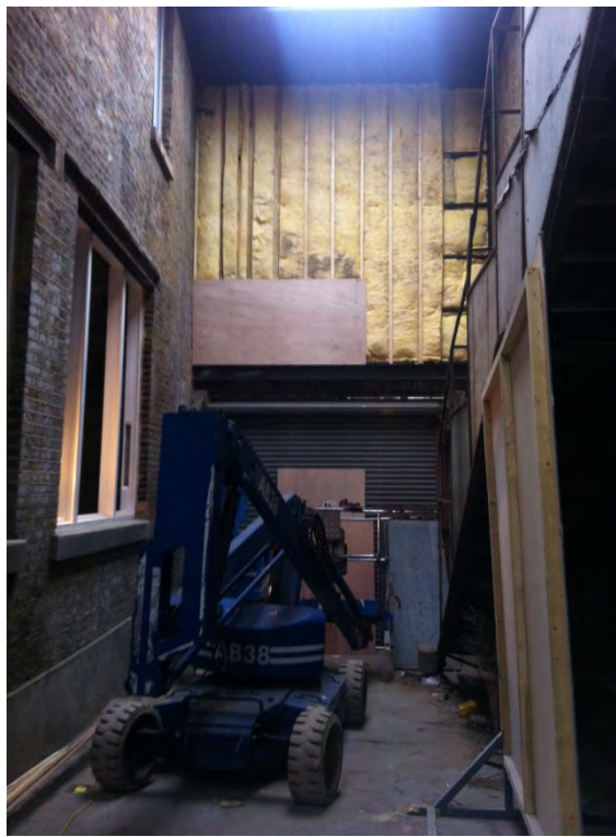
Internal elevation of Building facing Peck's Yard. This photograph shows (during installation) the second 100mm layer of rockwool installed behind the profiled metal sheeting. This also shows (during installation) the layer of 12mm plywood being installed behind the rockwool insulation.
