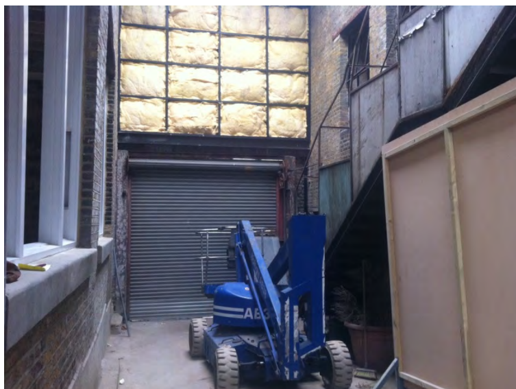
Internal elevation of Building facing Peck's Yard taken from the Atrium looking towards Peck's Yard. This photograph shows (during installation) the first 100mm layer of rockwool installed immediately behind the profiled metal sheeting.
