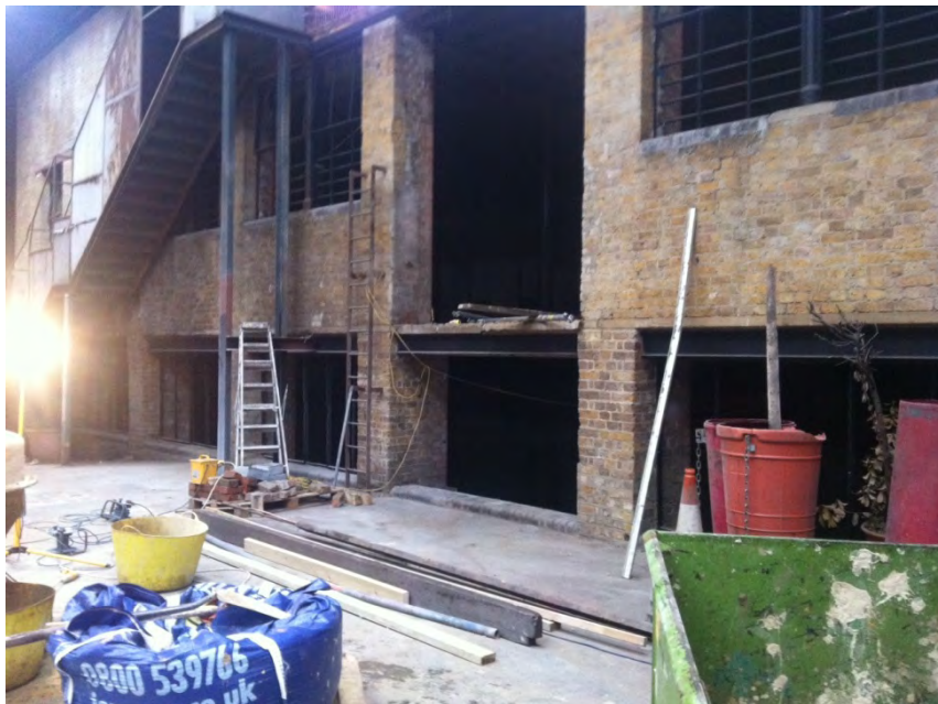
Openings between Gallery 1 and Atrium (to be reglazed as per drawings)
