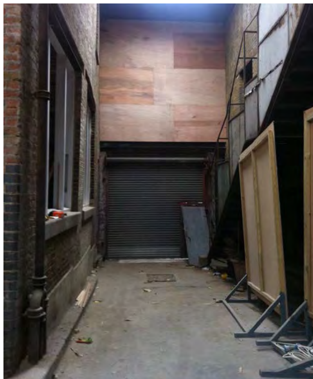
Internal elevation of Building facing Peck's Yard. This photograph shows (during installation) the second 100mm layer of rockwool installed behind the profiled metal sheeting. This also shows (during installation) the layer of 12mm plywood being installed behind the rockwool insulation.
